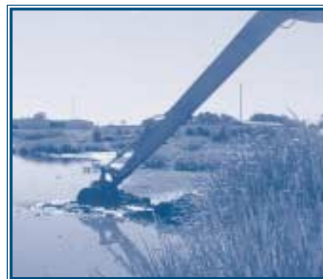
Silt removal from Brown Hill Creek in progress at Netley
