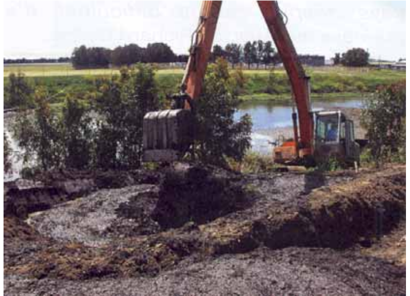
Around 30,000m 3 of contaminated silt trap material is built up in four Adelaide basins.
