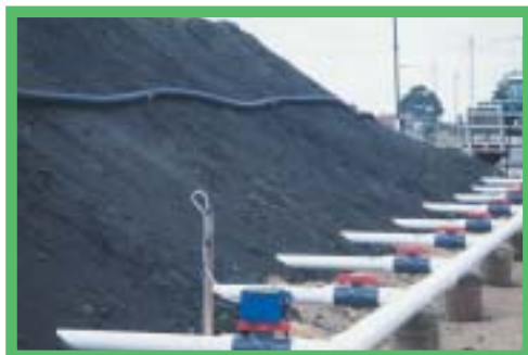
A forced aeration biopile for treating contaminated soil
