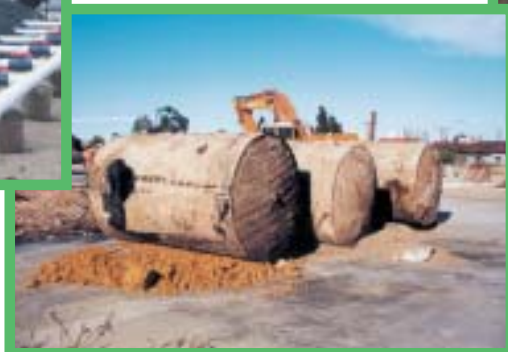
Excavation of underground fuel storage tanks and contaminated soil
